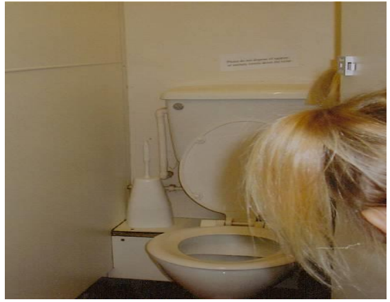
low level toilet
